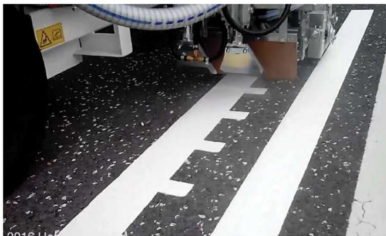
**PINTABANDAS CON DISEÑO MODULAR DE BASTIDOR
